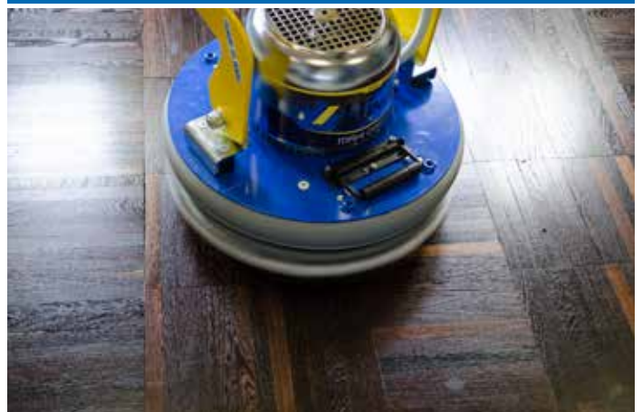
Oil finishing for parquet with raised wheels
