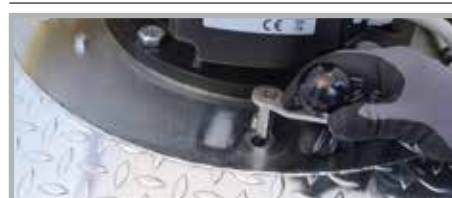
DCS System ON/OFF
