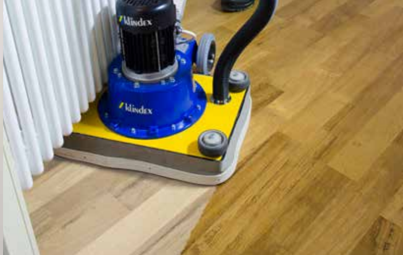
Works in tight spaces
