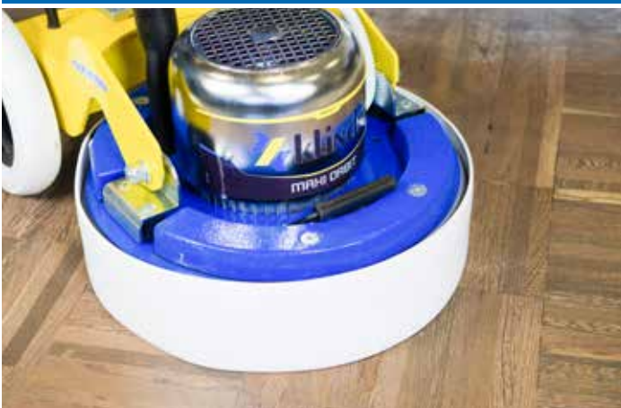
Grinding and sanding parquet
