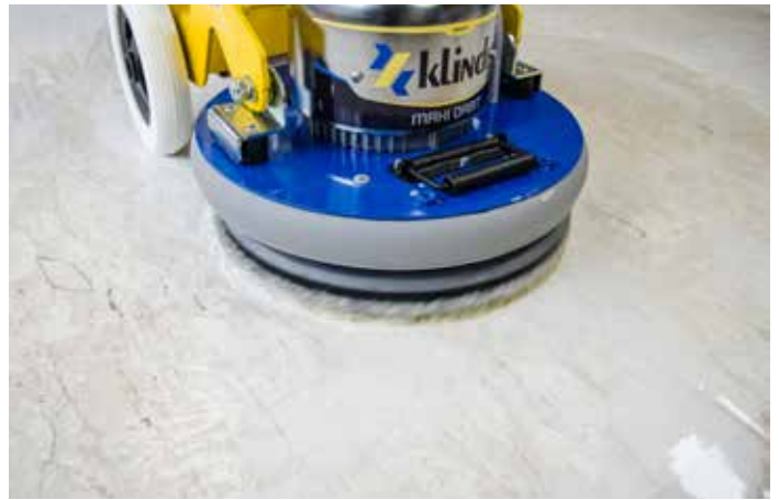
Micro-grinding of natural stone
