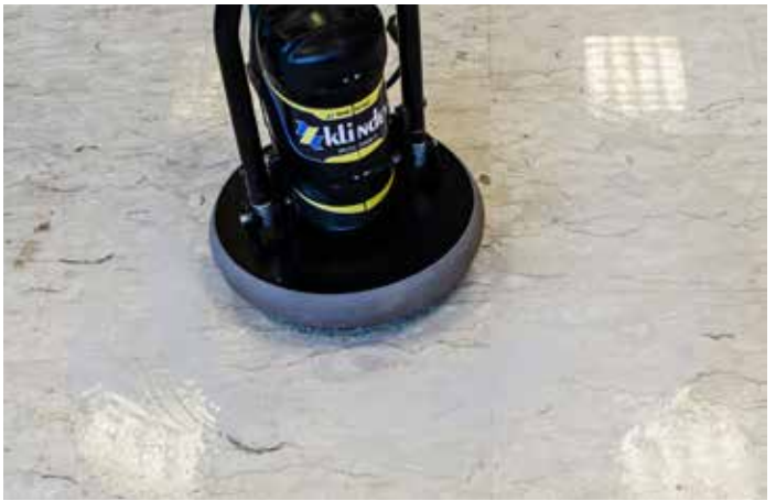
Micro-grinding of natural stone
