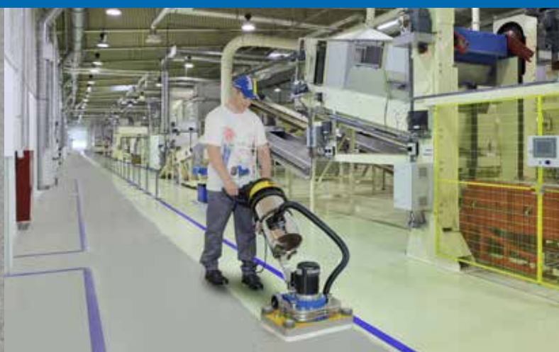
Restores and cleans resin and painted floors
