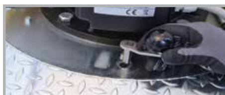
DCS System ON/OFF
