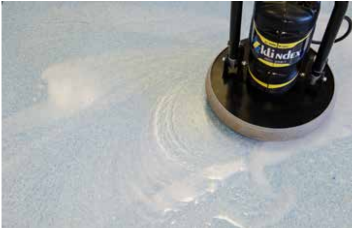
De-waxing linoleum, PVC and rubber
