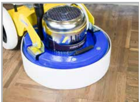
Grinding and sanding parquet
