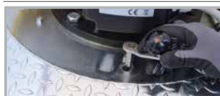
DCS System ON/OFF
